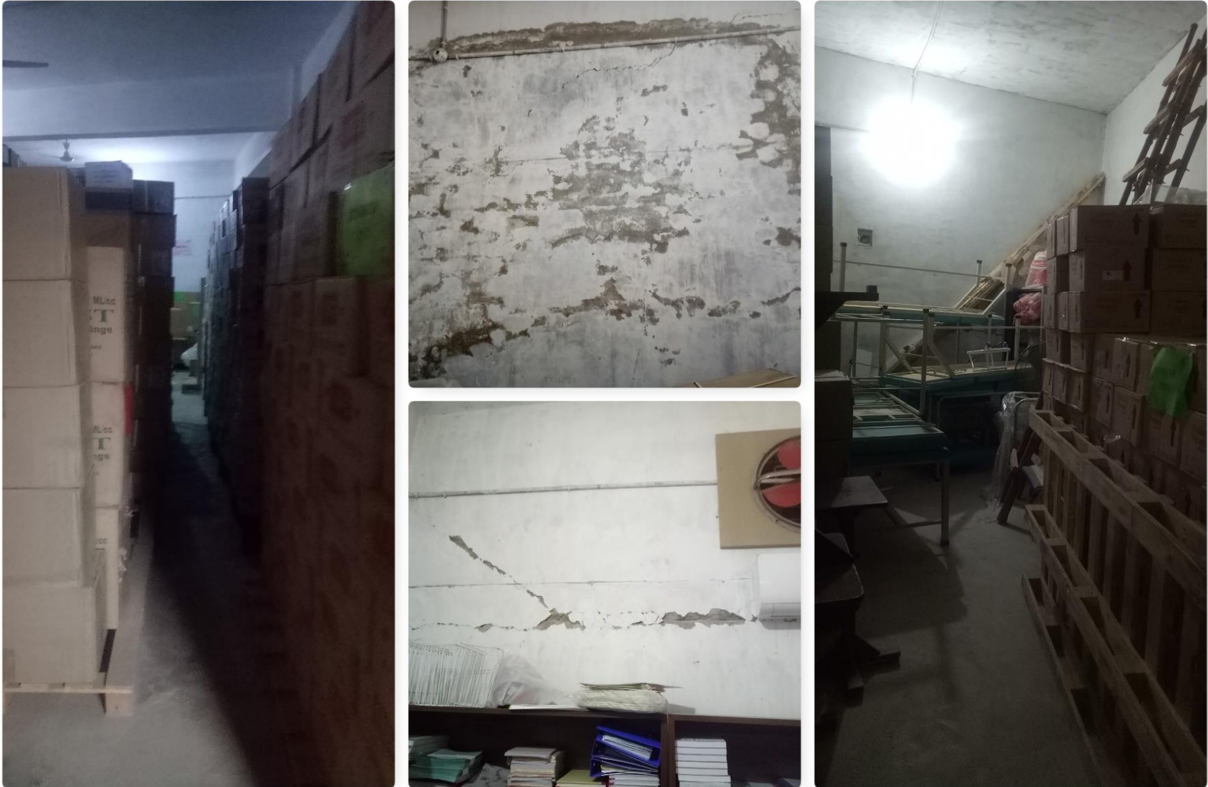
Figure 31: Snaps from the warehouse of district Sanghar B
